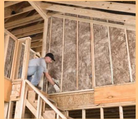
**EcoBatt Insulation is naturally brown—** assures no phenol, formaldehyde, acrylics or artificial colors are used in the manufacturing process.
